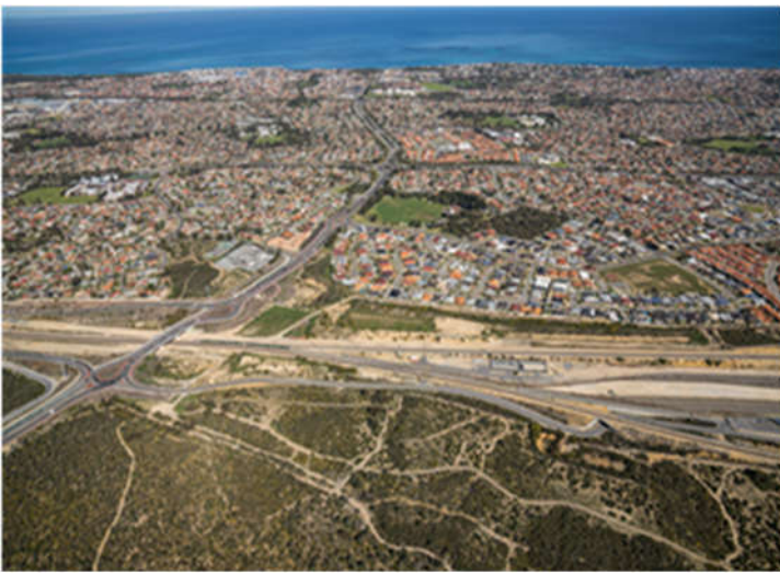
Figure 10: View West across current Hester Avenue Interchange
