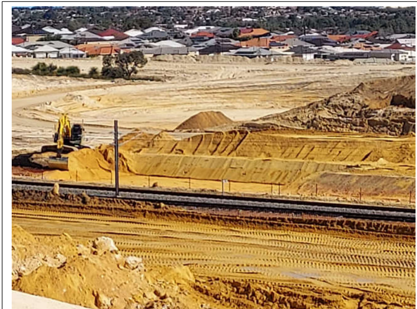
Figure 4: Cut to fill operations adjacent to Butler (Zone 1)
